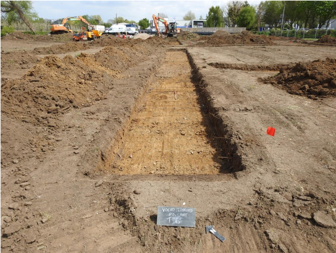
Plate 7: Trench 6 looking northeast, one-metre scale
